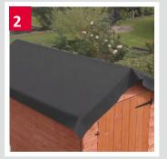
Relax the rubber membrane by laying it in position on the roof for at least 20 minutes.
