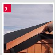
Trim the Rubber membrane back using scissors.
