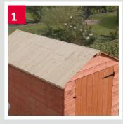
Remove the old roof covering and any nails. Replace the roof boarding if the roof is damaged of if the roofing felt does not come off.
