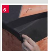
Replace any existing timber barge boards to help secure the membrane perimeter.
