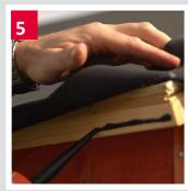
Apply edge sealant using a mastic gun to the roof edges. Once dried this will hold the membrane securely.
