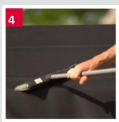
Put membrane on and sweep down to ensure all trapped air bubbles are removed and membrane bonds to the adhesive.
