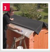
Apply the adhesive working from the centre of the roof outwards in stages. DO NOT let the adhesive dry out.
