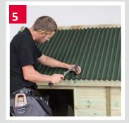
Place the next sheet onto the first with a two corrugation overlap and fix as before.
