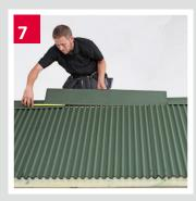
Place the ridge pieces on the top of the roof and overlap to ensure they extend from one end to the other, if necessary covering any existing timber barge boards.
