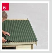
Fix the final sheet next to the second with the appropriate overlap and ensure that it aligns with the edge of your shed roof and then nail.
