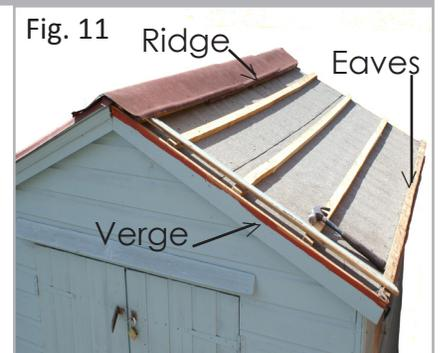
**Fixing battens to thin decks: (Fig. 9 & 11).** To secure battens onto an existing thin roof decks, first nail the battens in position at the verges from above, then mark and screw the battens in place from inside the building.
